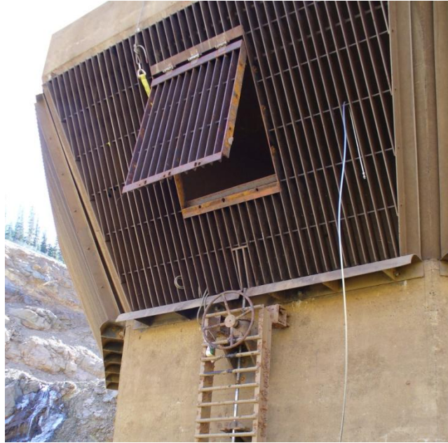
Figure 3. Upper reservoir mushroom access hatch
