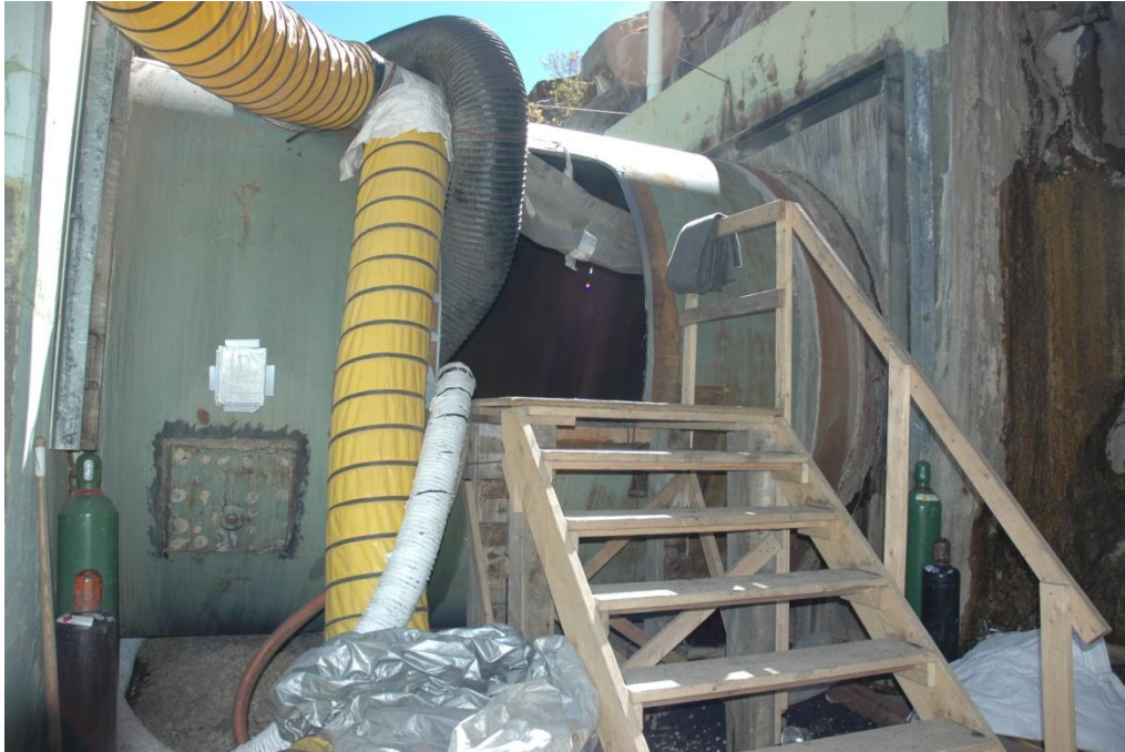
Figure 4. Access door cut into penstock for recoating work
